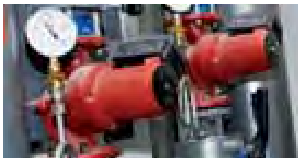
Actuators, valves, control cabinets
